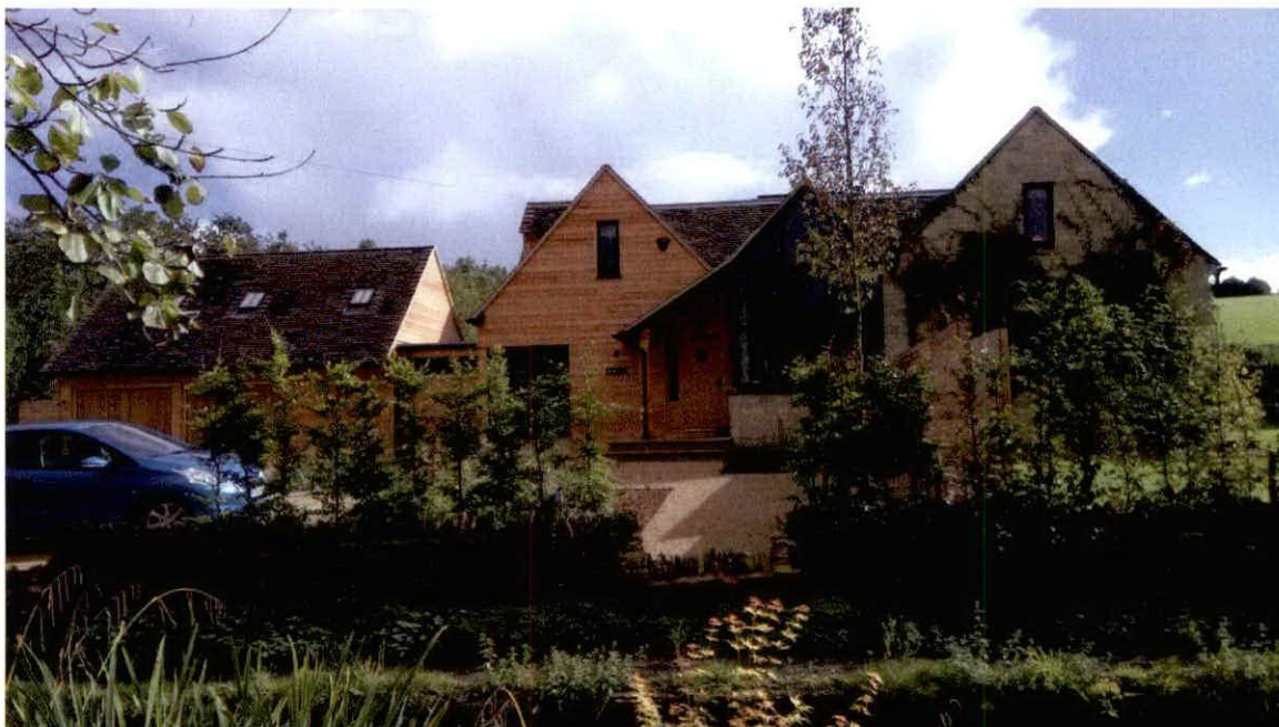
Photograph 1 Current View of Close Hill from Hatters Cottage rear patio
